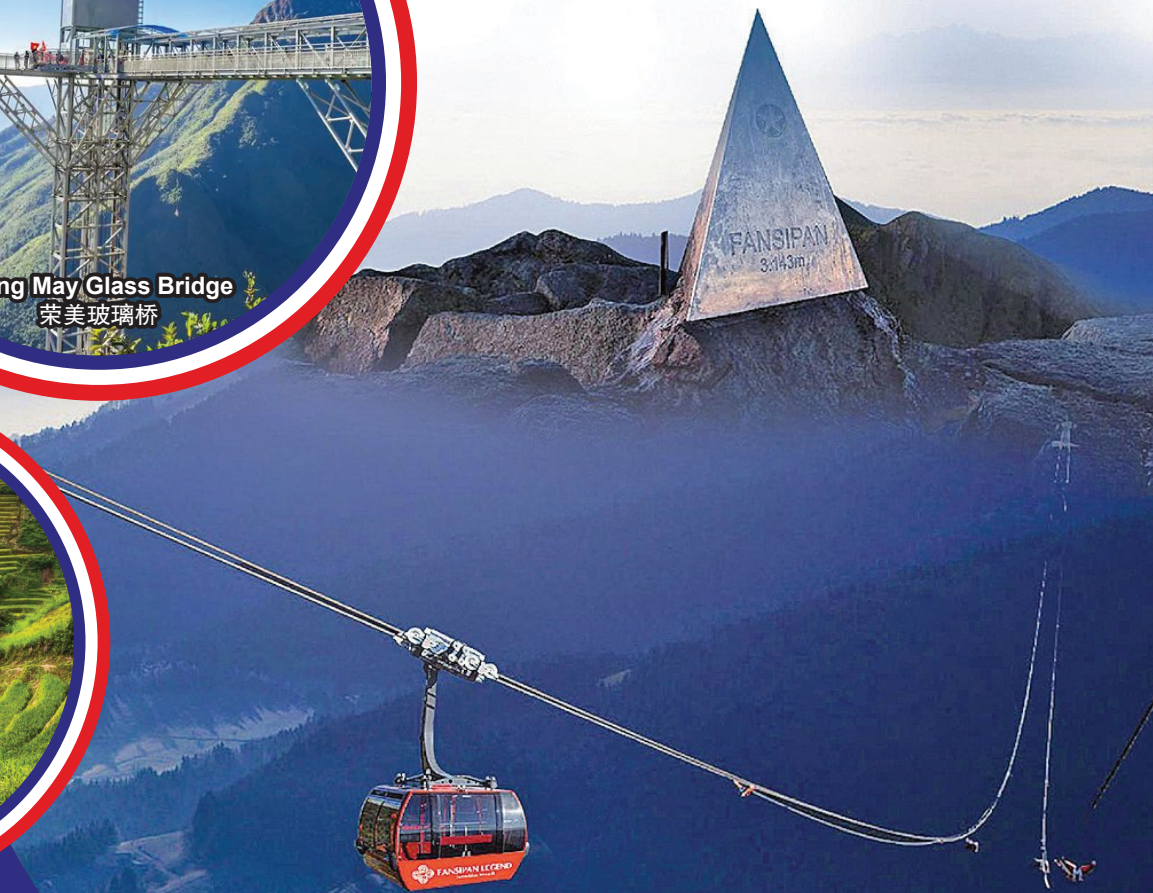
Mt. Fansipan Cable Car 番西邦峰缆车
